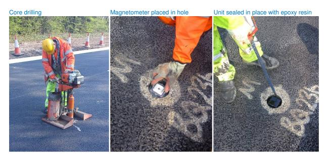
Although these units were installed whilst the sections of road were closed, it proved that they can be fitted in a much quicker time than a traditional inductive loop, and that because they are positioned in the centre 272973/HWY/TTS/001/A 20 September 2011
